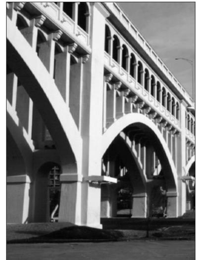
Products are often applied by spray equipment. Here material had to be roller applied because of wind, the proximity to the Cuyahoga River and vehicular and pedestrian traffic that continued under the bridge during painting.
