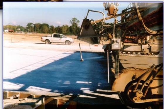
With the concrete poured and finished, Safe-Cure 2000 curing compound is spray applied at 150 - 200 square feet per gallon. It helps the concrete achieve its maximum impact and abrasion resistance while reducing shrinkage cracking.
