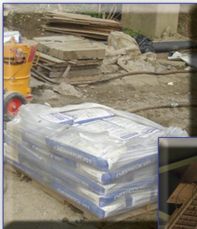
**ChemPatch VO1** was placed in one application averaging 2.5 inches deep. Finishing the surface with a currycomb (serrated metal horse comb) completed the project.
