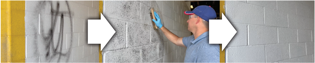
Graffiti Eraser removes graffiti from substrates coated with Graffiti Stopper.
